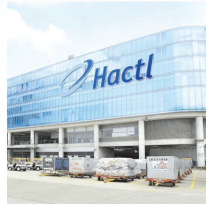
■ Exterior of Hactl building
